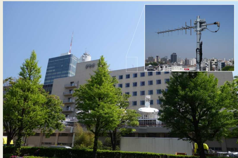
Reception Antenna @NHK Broadcasting Center
